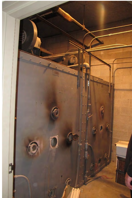
Fig. 48 – Interior, lower level, original crematorium equipment (no longer in use).
