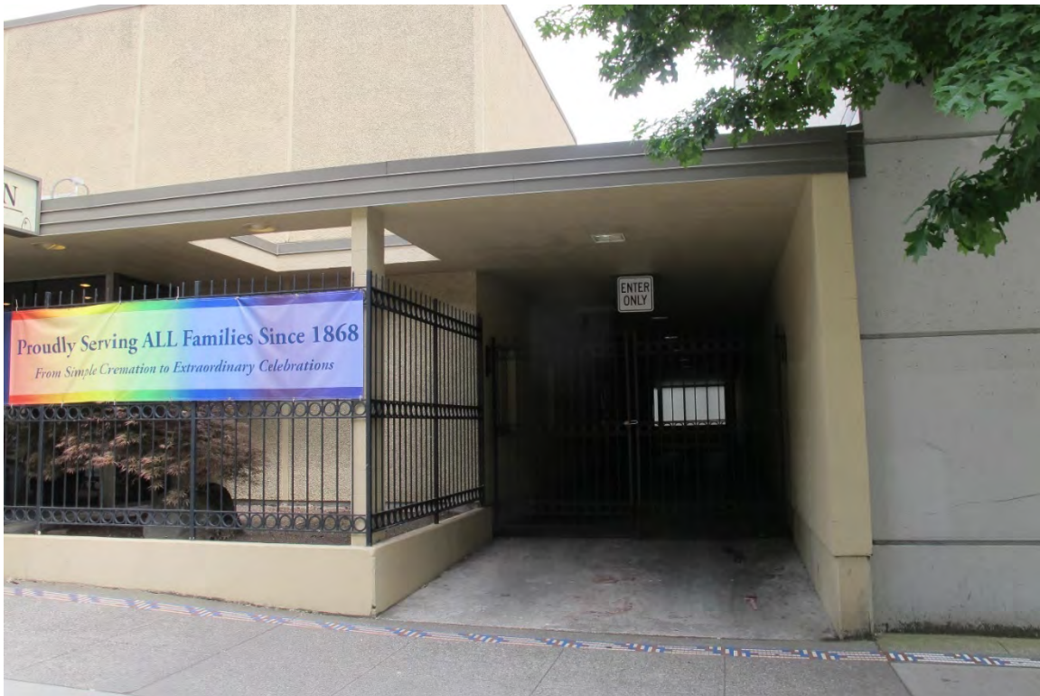
Fig. 26 – West or front elevation, detail of perimeter driveway entrance.
