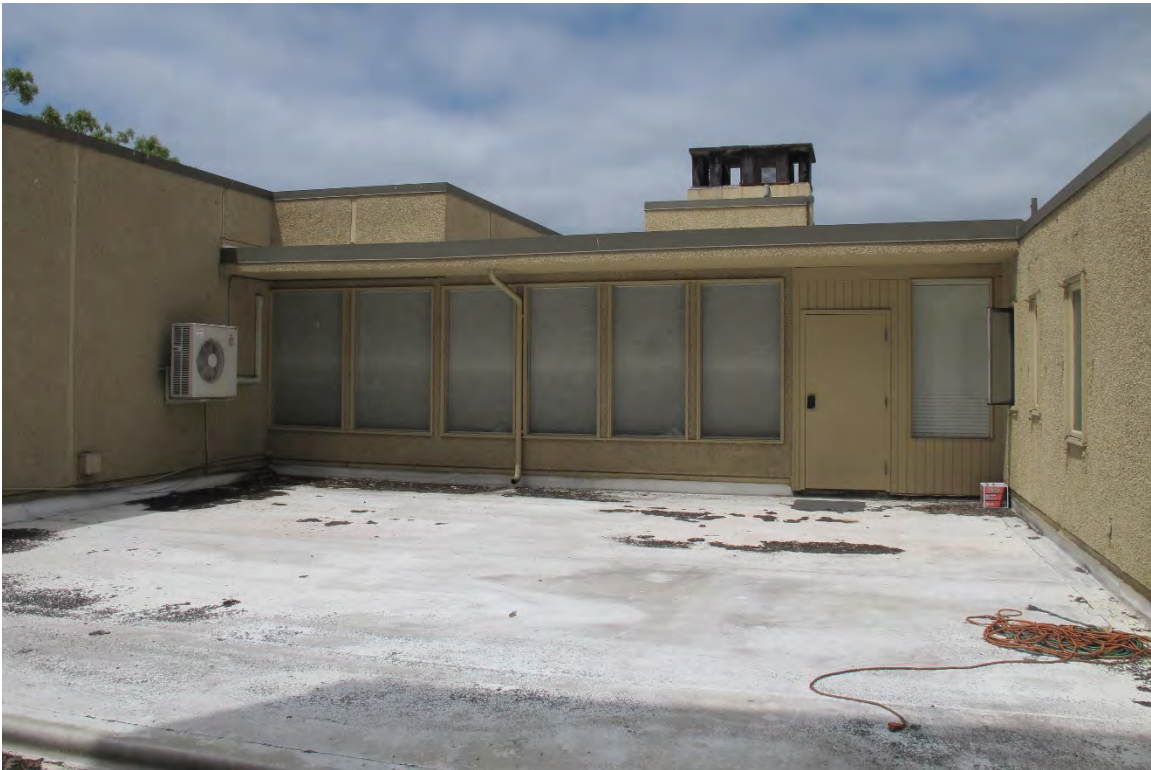
Fig. 56 – Roof, center part of building, view towards interior of parcel.
