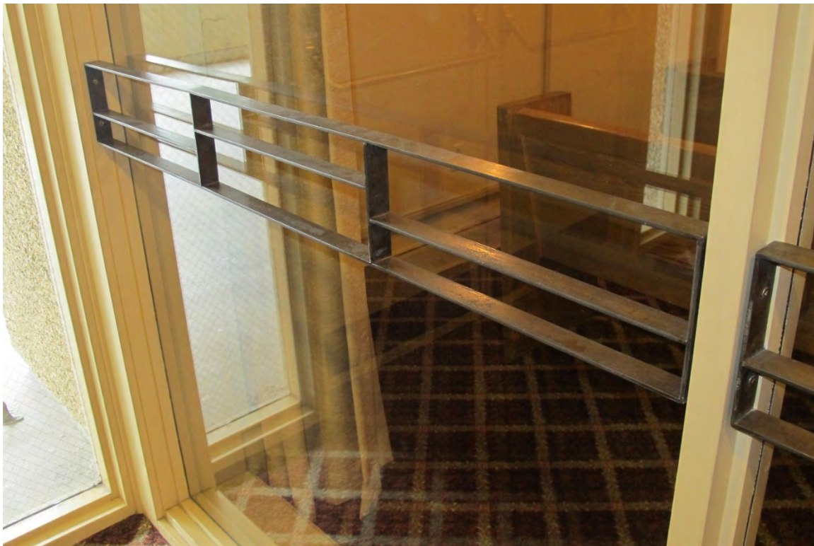
Fig. 36 – Interior, railing on hallway side of main chapel glazing.
