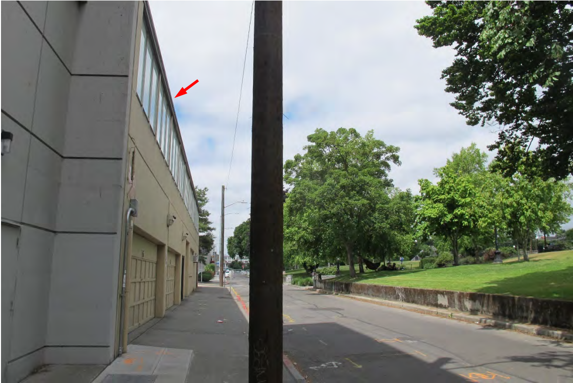
Fig. 14 – View northward on Nagle Place; subject building indicated by arrow. Cal Anderson Park visible at right.
