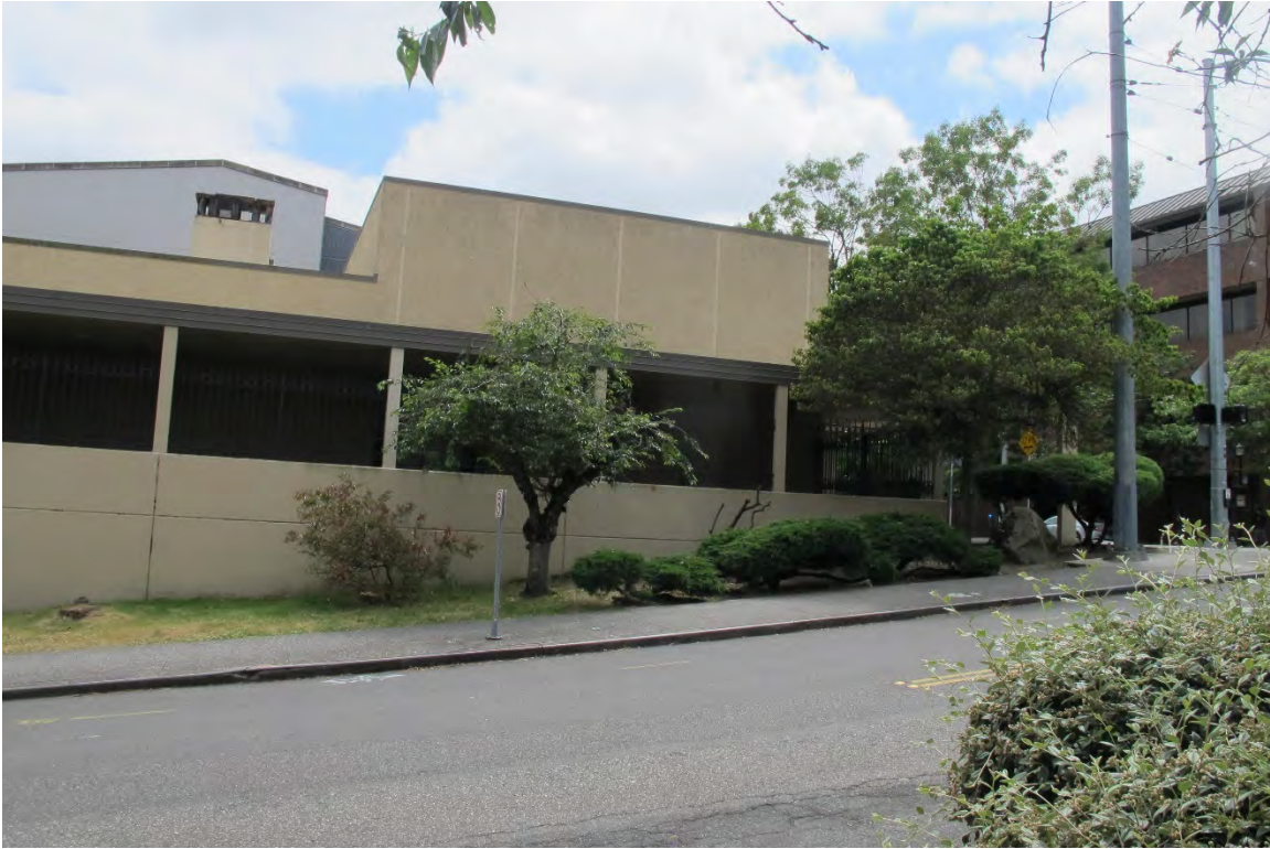
Fig. 11 – North or side elevation, facing East Howell Street.
