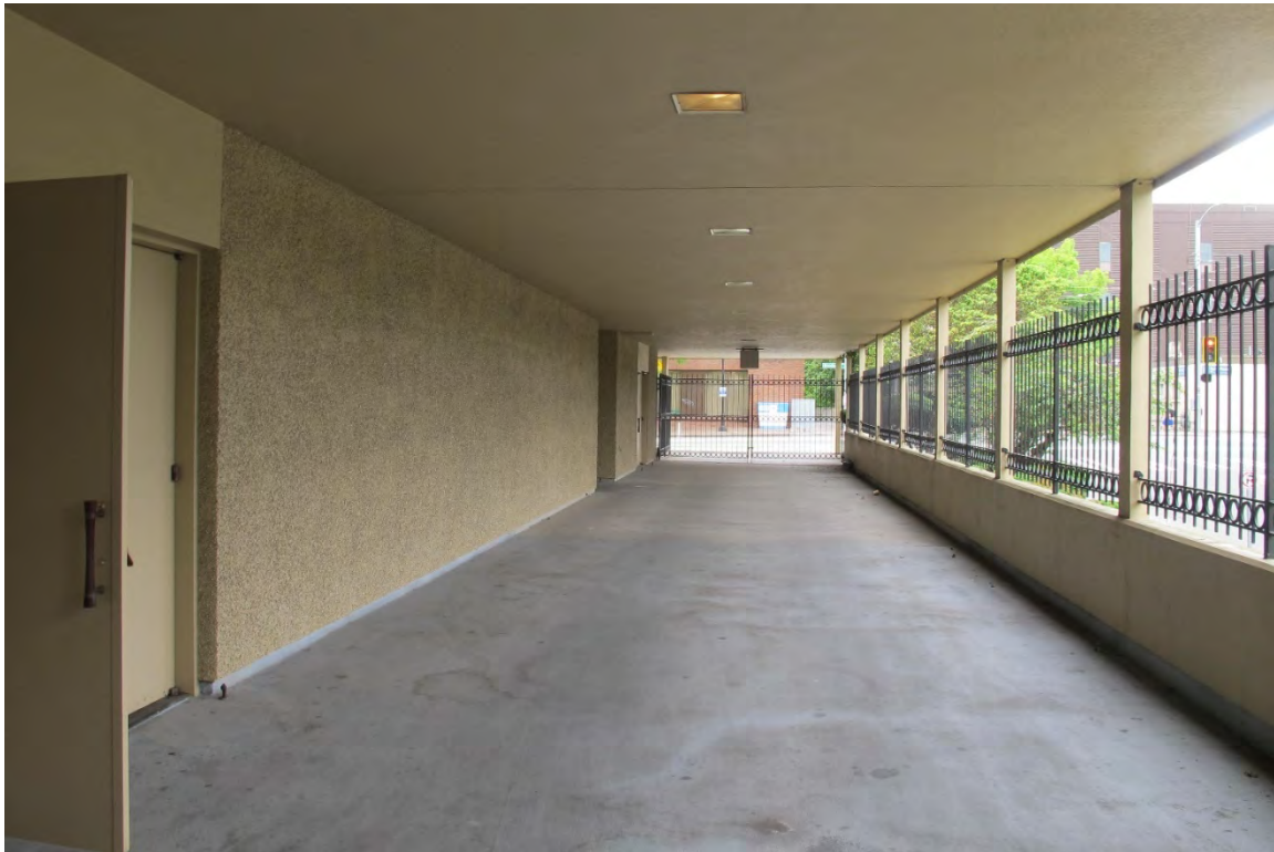
Fig. 28 – Perimeter driveway at north side of building, view westward towards Broadway.
