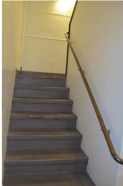
Fig. 46 – Interior, typical stair.
