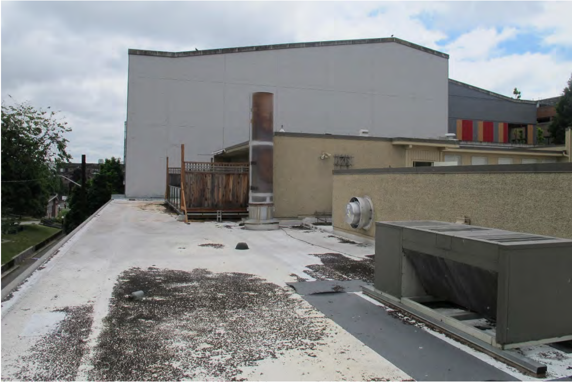
Fig. 53 – Roof, east edge, view southward. Tall wall in distance is part of adjacent Seattle Central College structure. Wood fence is part of subject building's upstairs apartment exterior space.
