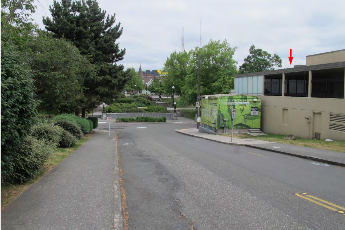
Fig. 13 – Context: View eastward on East Howell Street; subject building indicated by arrow.
