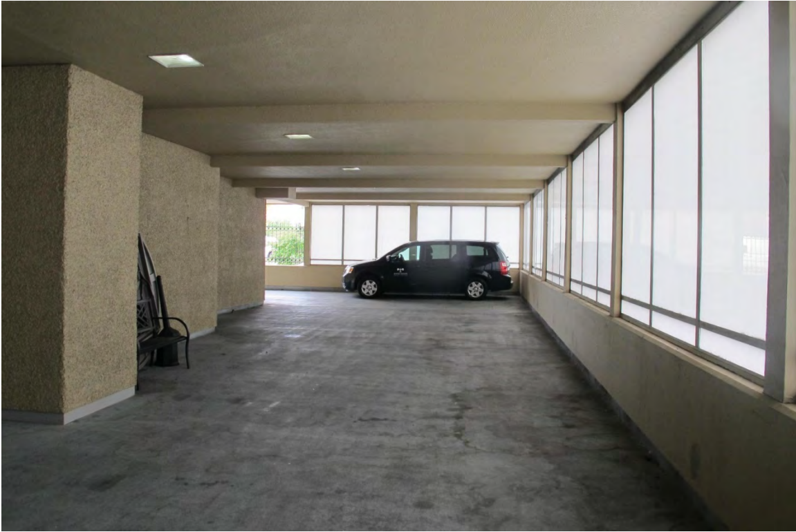
Fig. 29 – Perimeter driveway at east side or rear of building, view northward.
