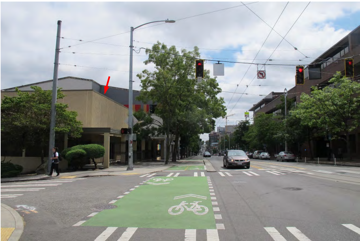
Fig. 20 – Context: View southward on Broadway; subject building indicated by arrow.
