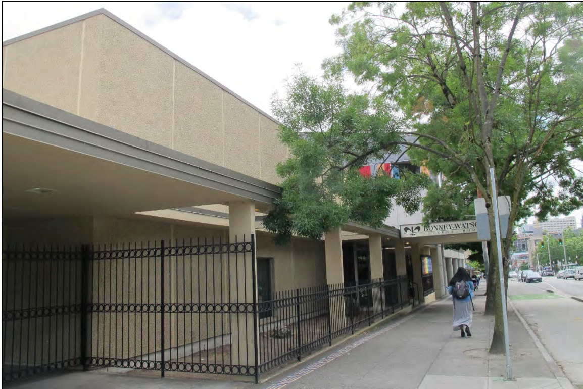
Fig. 21 – View southward on Broadway in front of subject building. Black metal fencing is non-original.
