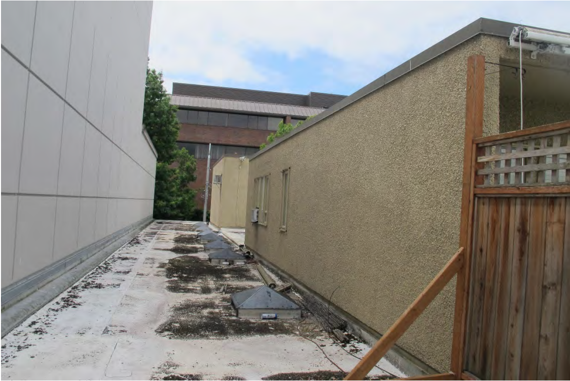
Fig. 55 – Roof, south edge, view westward towards Broadway. Perimeter driveway is below.
