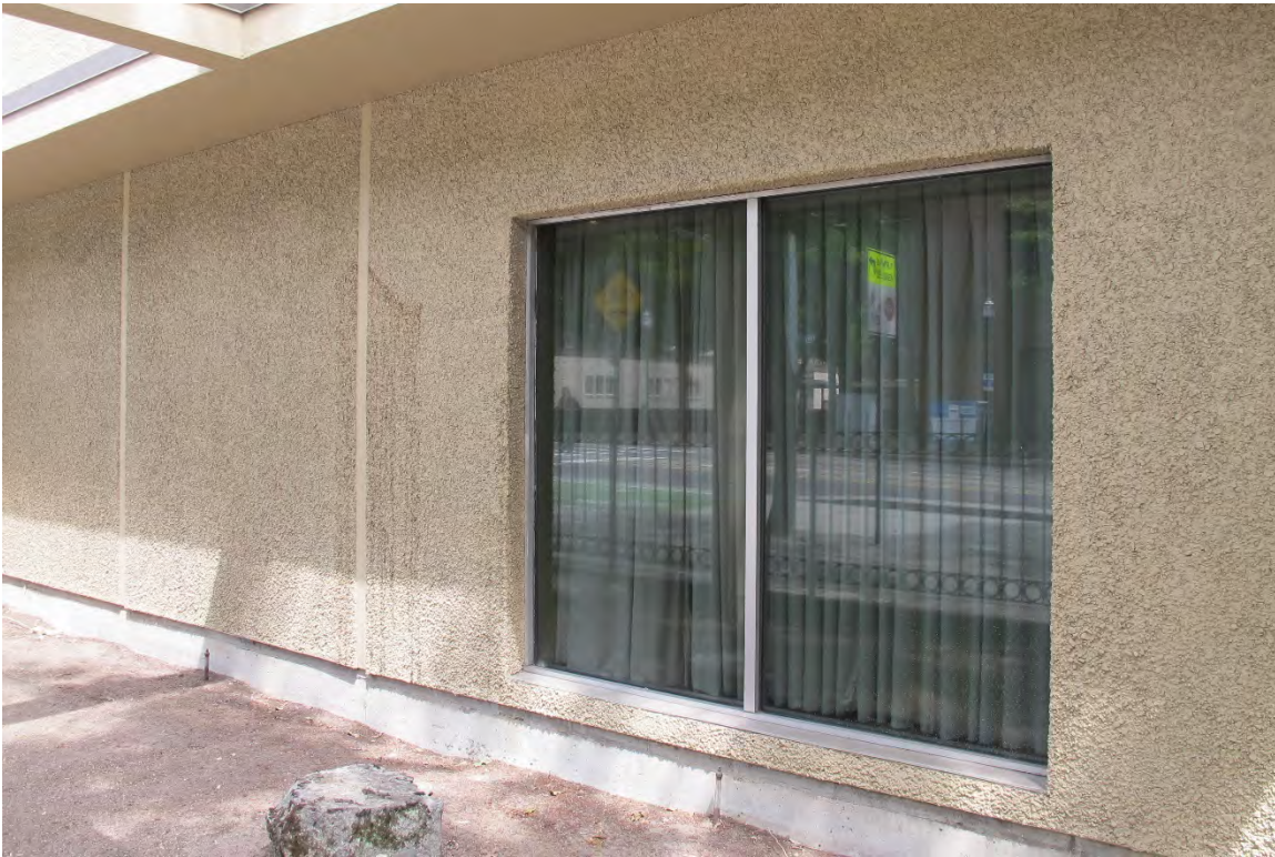
Fig. 24 – West or front elevation, detail of covered garden area, marblecrete wall, window.
