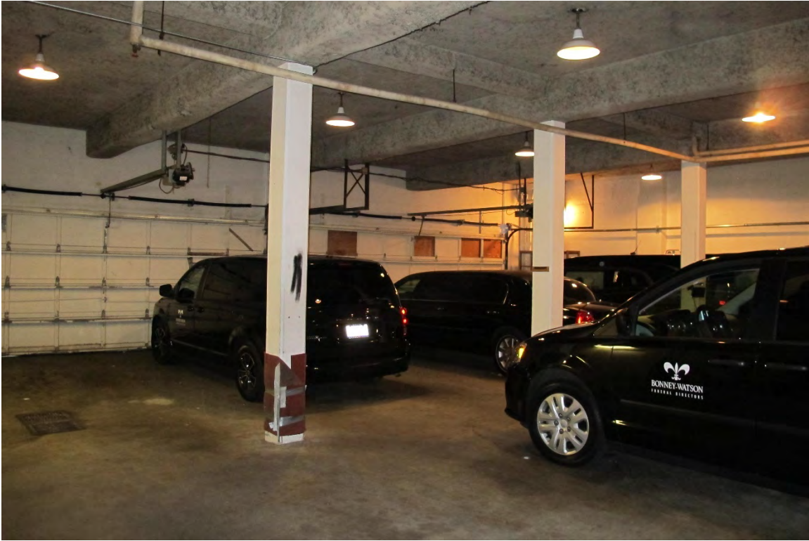
Fig. 49 – Interior, lower level garage.
