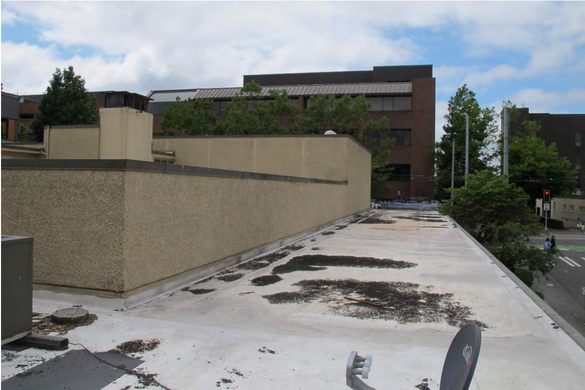
Fig. 54 – Roof, north edge, view westward towards Broadway. Perimeter driveway is below.
