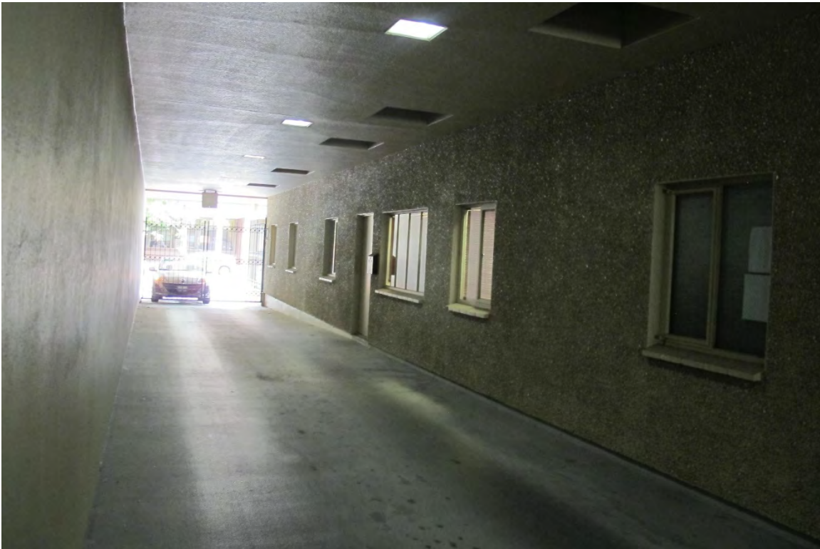
Fig. 30 – Perimeter driveway at south side of building, view westward towards Broadway.
