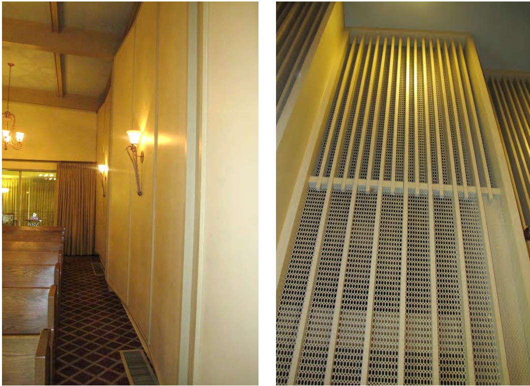
Fig. 39 – Interior, main chapel, detail of side wall showing angled panels (left); and wall screen at front (right).
