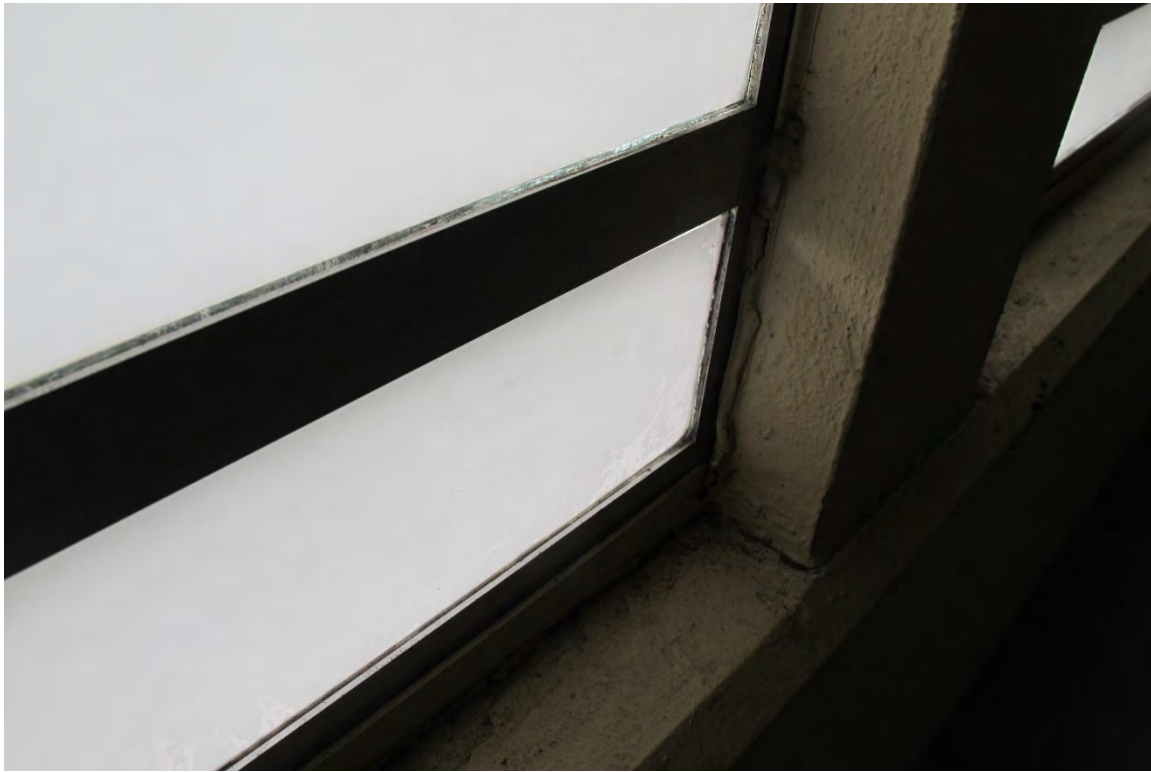
Fig. 31 – Perimeter driveway at east side or rear of building, detail of glazing.
