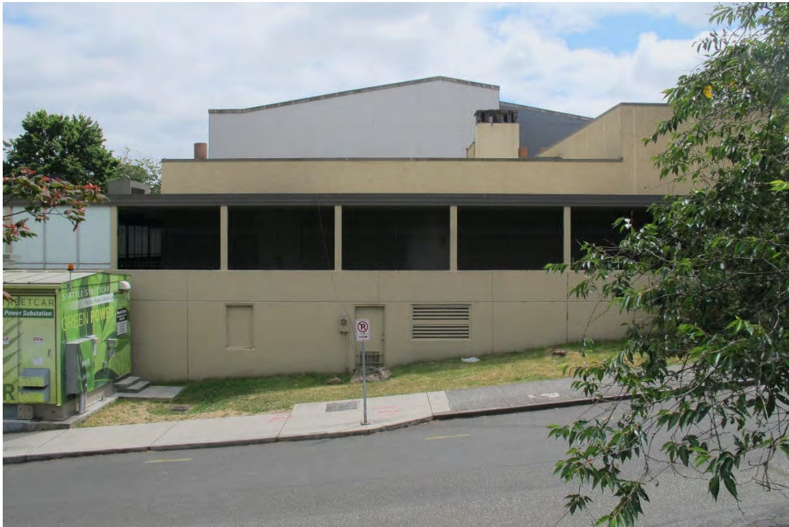
Fig. 8 – North or side elevation, facing East Howell Street.
